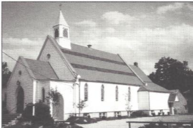
915 Vine Avenue, formerly the New Covenant Gospel Church, is now housing apartments and has a completely renovated interior and exterior.
